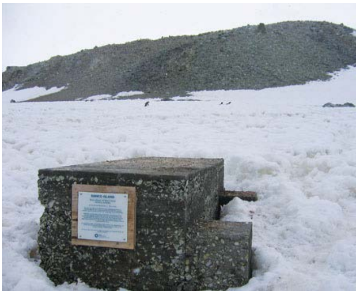
The site of the former British base is marked with concrete foundation blocks.
